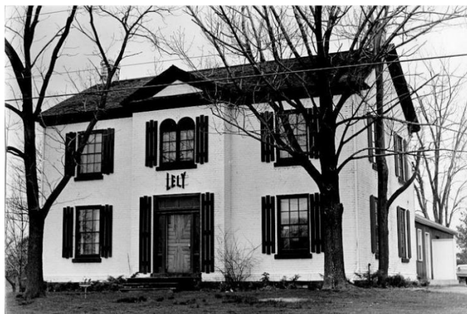
5355 North Service Road
